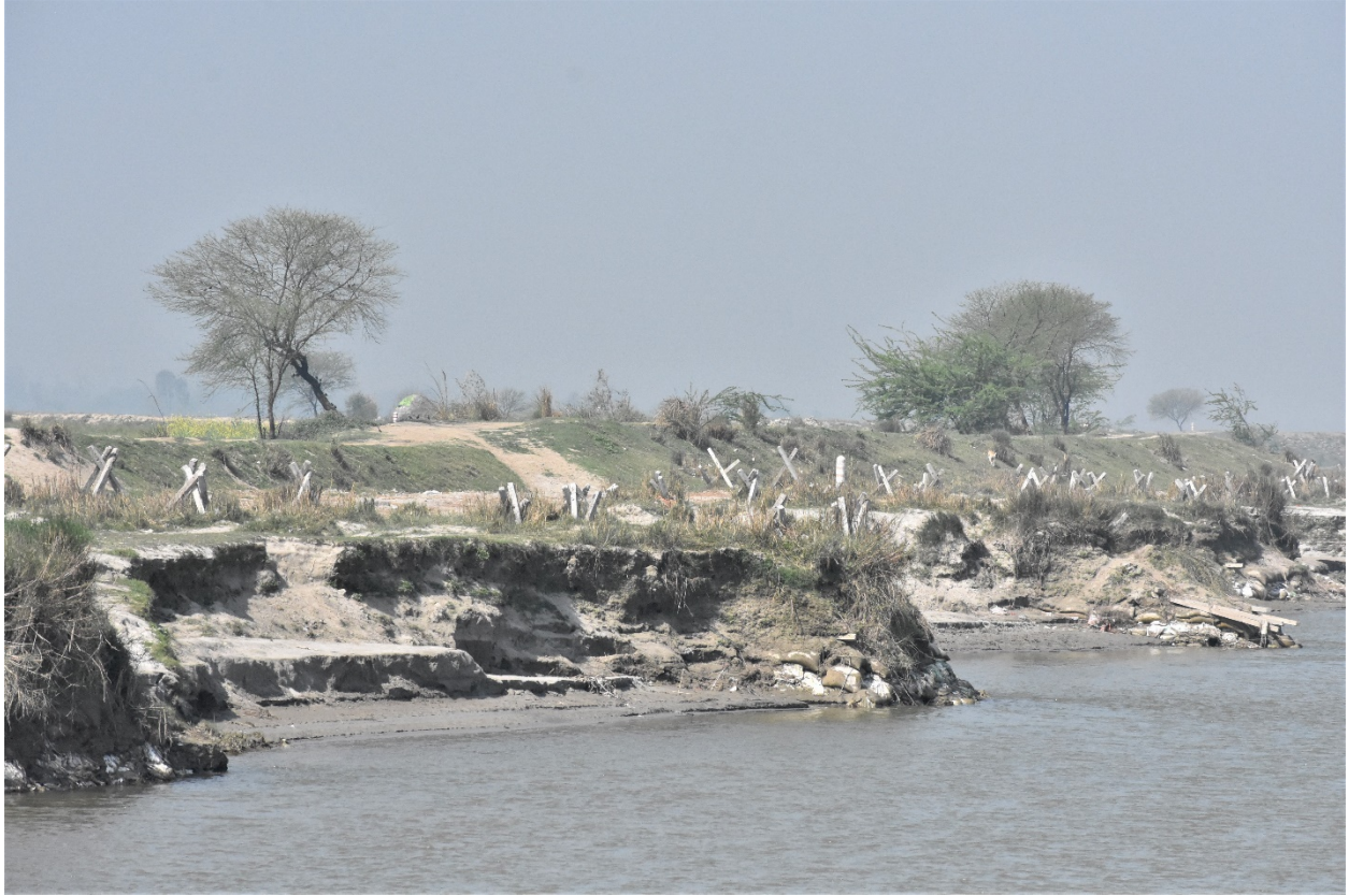
Image 31 : Ganga River Bank Erosion As Observed Near Kadarganj Ghat In Kasganj Distt.
